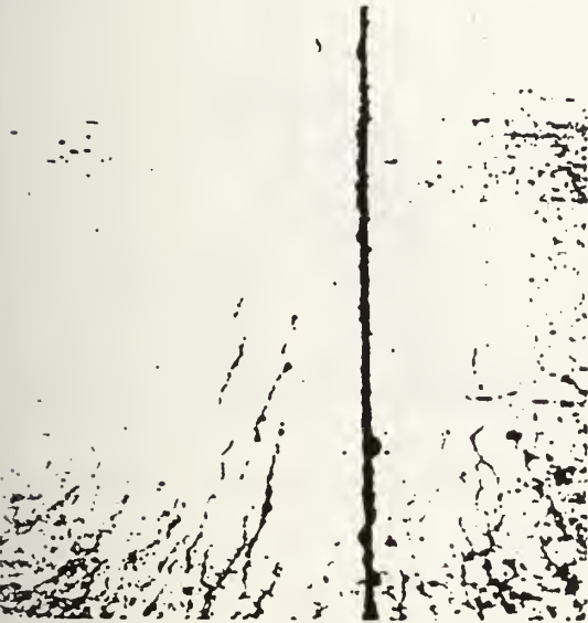
Fig. 3.2.4.4 — D-cracking
